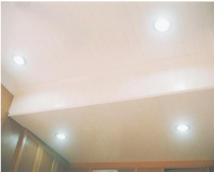
MADE OF 'ACCUCEL' RIGID PVC FOAM PROFILE WITH INTEGRAL SKIN
